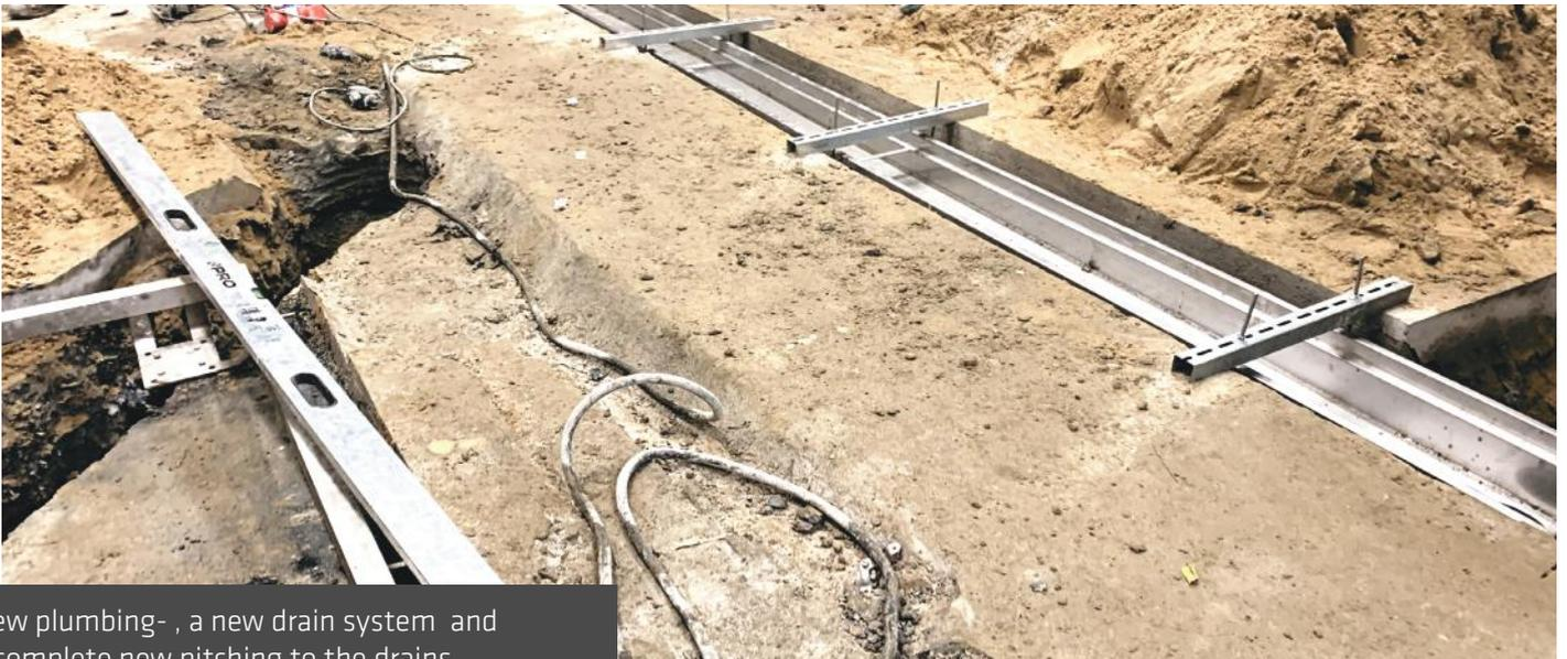
New plumbing- , a new drain system and a complete new pitching to the drains
