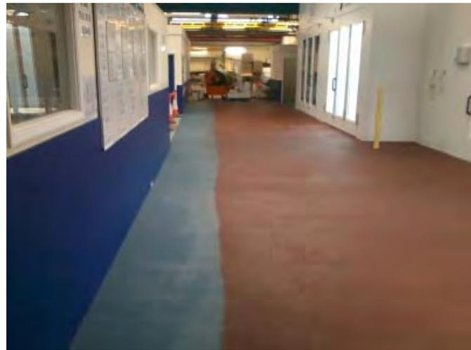
Due to the nature of the works that take place within the facility, the client requested areas to be demarcated to maintain a safe working environment. This was achieved in the first instance by the installation of different colours of our Stonclad GS mortar.
