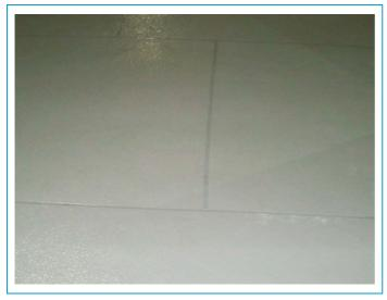
Following installation of the Stonclad system, all construction joints were treated with Stonflex MP7. This heat resisting polyurethane sealant will allow for any movement within the expansion/construction joint within the new production area.
