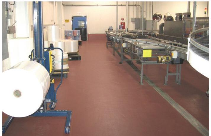
*Stonclad UT replaced an unsafe, failing epoxy floor in Cold Springs Brewery’s batching rooms.*
