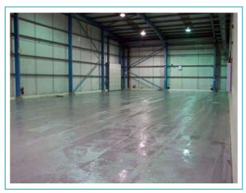
HT Primer laid 24 hours previously receives the Stonproof RH7 to provide a barrier between the cracked substrate and the finished epoxy floor.
